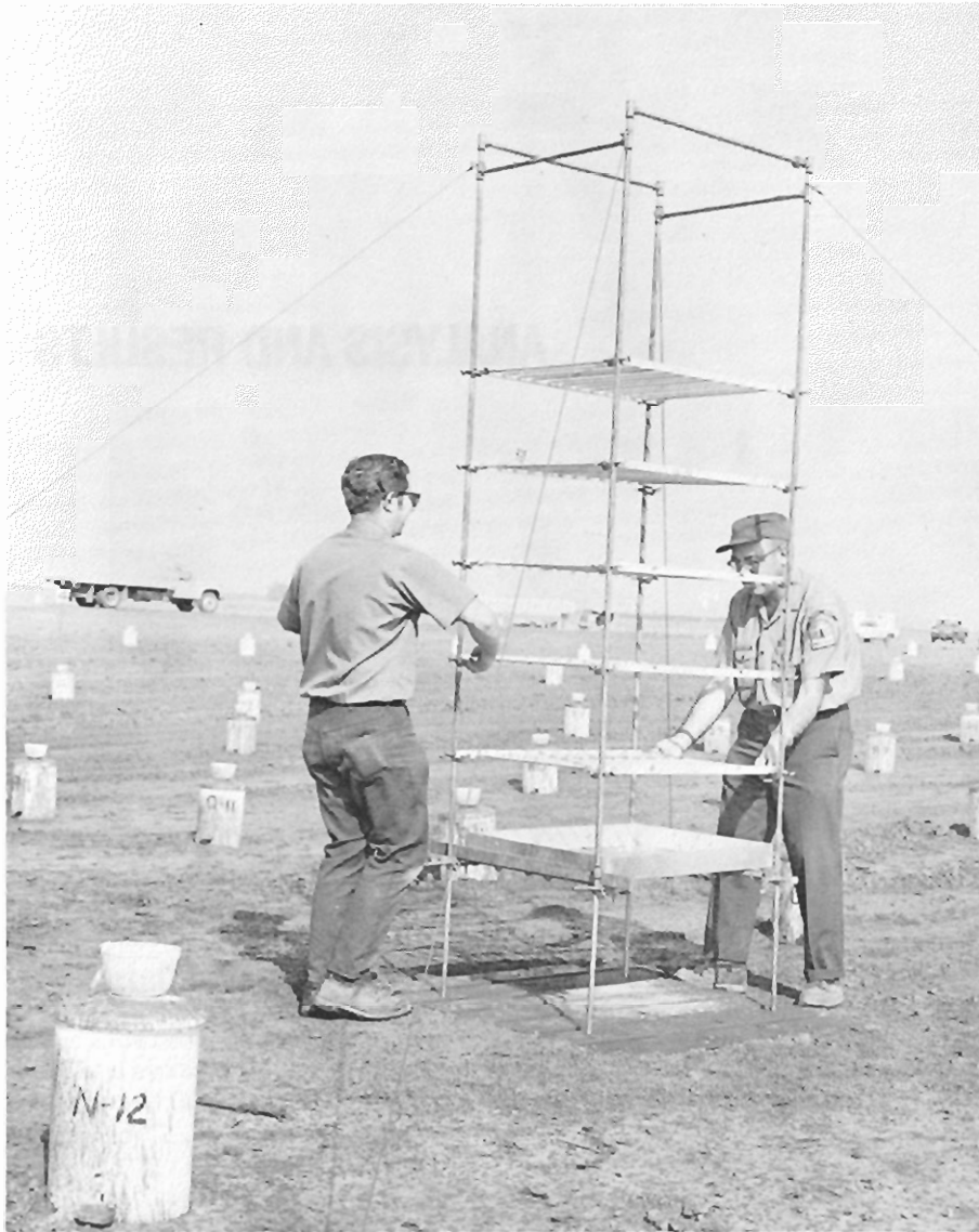
Figure 13.--Model used to measure the vertical distribution and retention of retardant.
